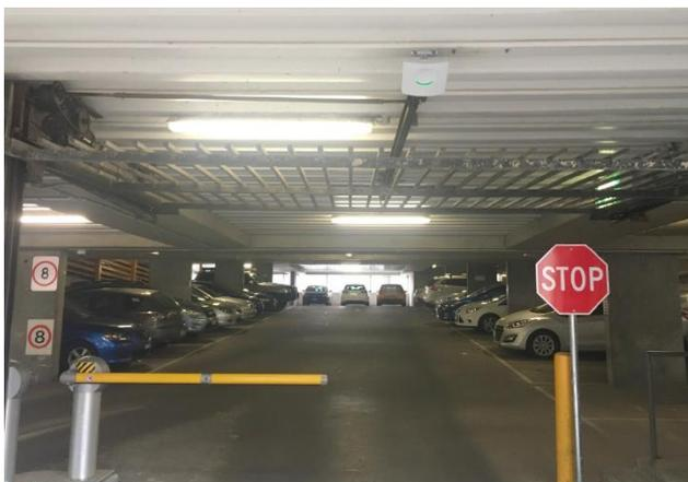
A [UHF Windshield Tag](#) that contains a unique identification number is adhered to the windshield of all staff vehicles. [uPASS Reach](#) readers installed at the 2 entry lanes and 2 exit lanes allow consistent reading of up to 5 meters. Based on UHF (Ultra High Frequency) technology, these readers offer the right solution for straightforward access to car parks of hospitals, campuses, gated communities, etc.
